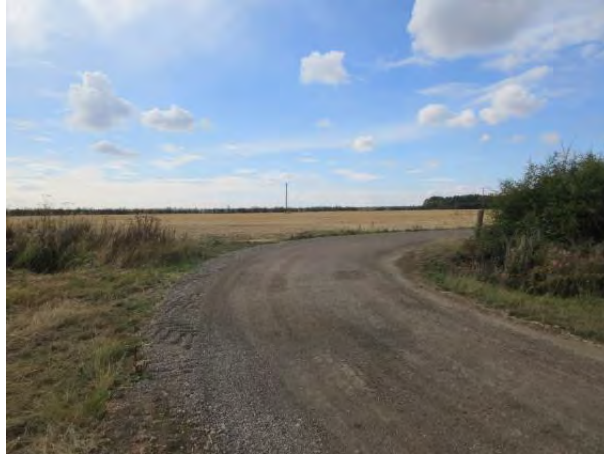
Photograph 4 First right hand bend on farm track. Load moves away from camera. Negotiable. Temporary road widening via plates or hardcore could be undertaken if required to widen road surface but this is not expected to be necessary.
